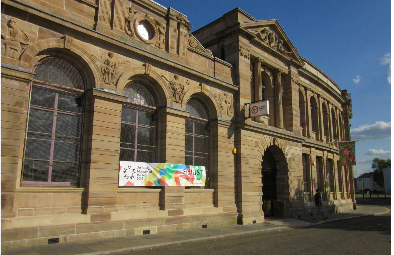
Glasgow Women's Library, dışarıdan görünüm. Glasgow Women's Library, an exterior view.
